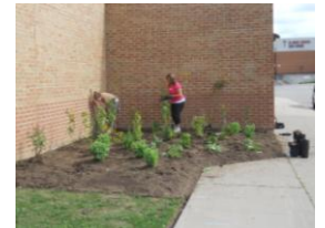
Installing a pollinator garden at St John school.
